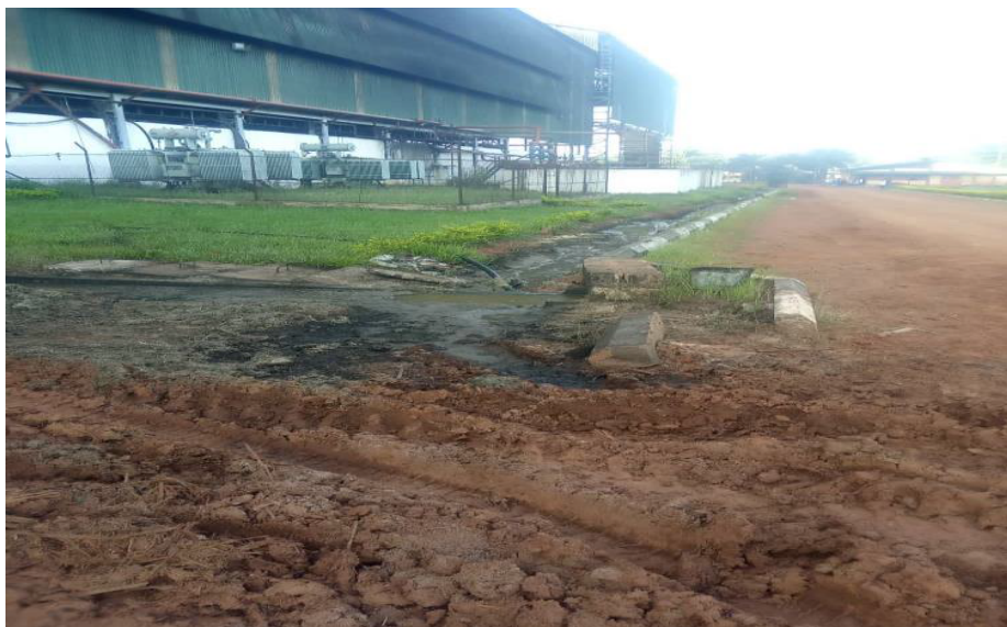
Photo 3: Open discharge of wastes before establishment of the ETP at Mayuge Sugar Factory.
