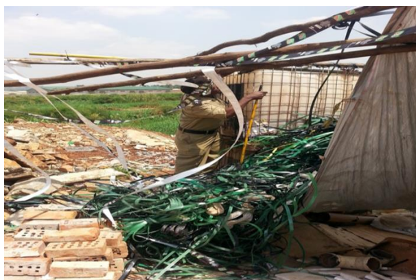
Photo 10- 12: EPPU destroying upcoming temporary structure in kinawataka wetland
