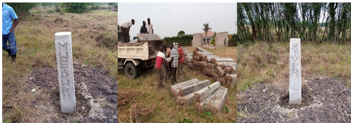
Photo 9- 5: Concrete pillars installed to mark the boundaries of buffer zone along River Rufuha in Rweikiro and Ngoma sub-counties
