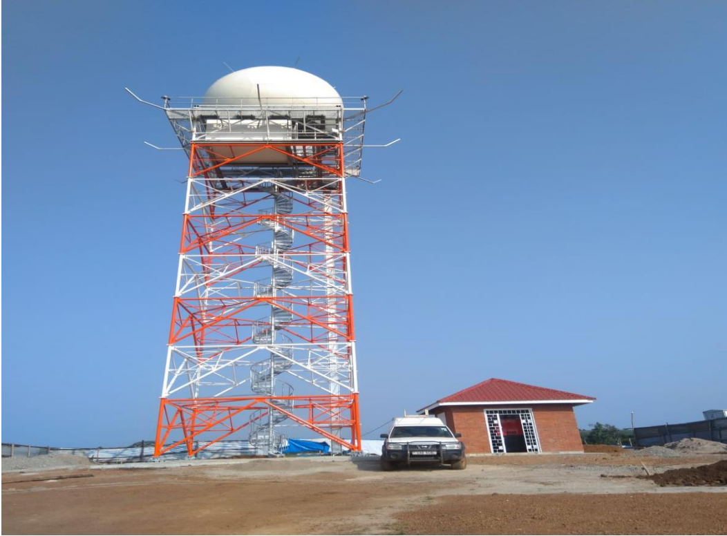
Photo 10- 35: First weather radar fully installed and operational in Kigungu
