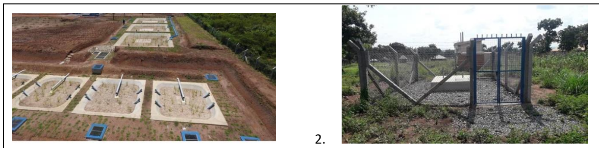
Photo 7- 1: Dzaipi FSTP (after construction). Photo 7- 2: Sludge Holding Tank in Nyumanzi
