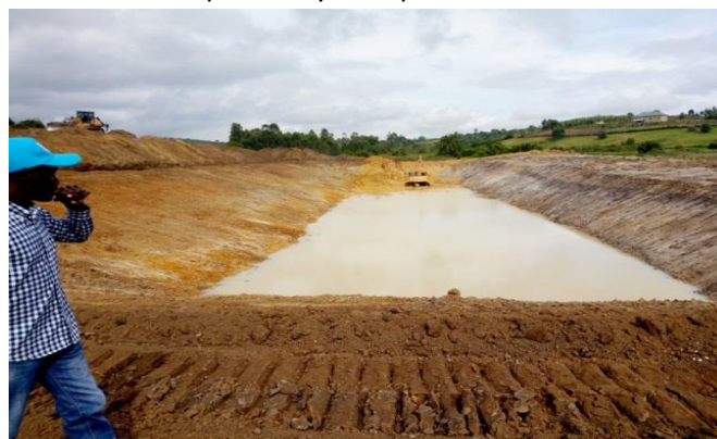
Photo 10- 10: Water retention facility for enhancing wetland recovery
