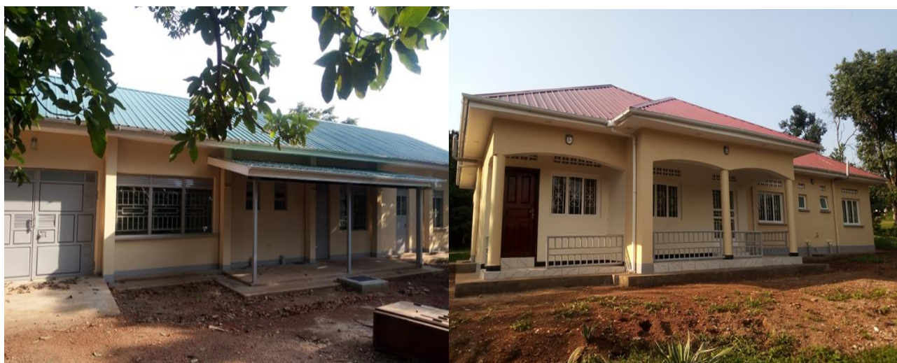
Photo 10- 22: Renovated staff quarters at Nyabyeya College
