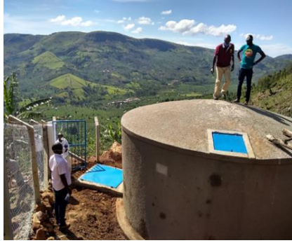
Photo12- 5: The 30,000 Litre reservoir tank - serves the upper line
