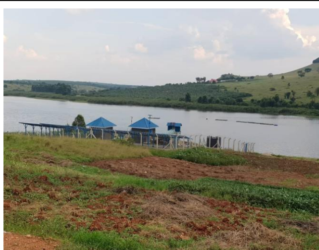
Photo 8- 1: Mabira earth dam in Mbarara District
