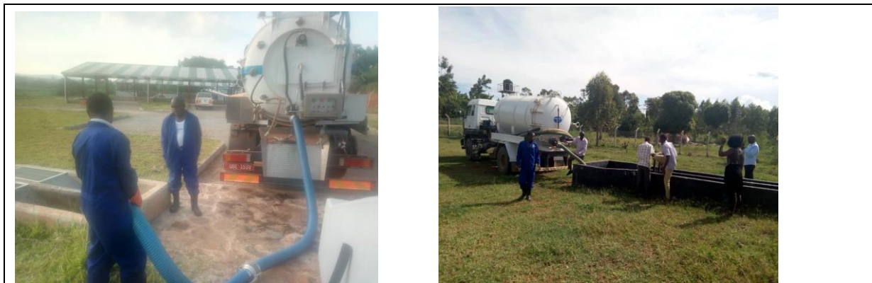
Photo 7- 5: Cesspool truck emptying sludge at Kiboga FSTP. Photo 7- 6: Cesspool Truck emptying sludge at Kayunga FSTP
