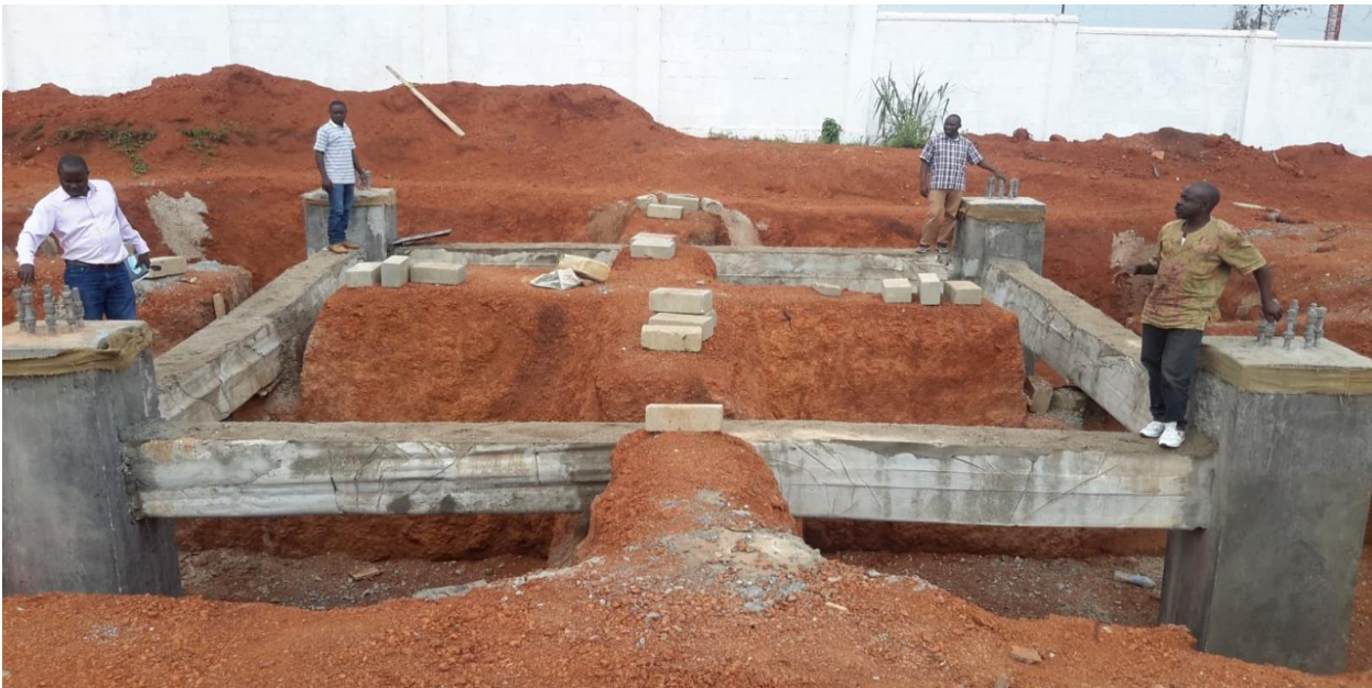
Photo 10- 36: Radar tower works for the second weather radar at Mwizi hill in Rwampara
