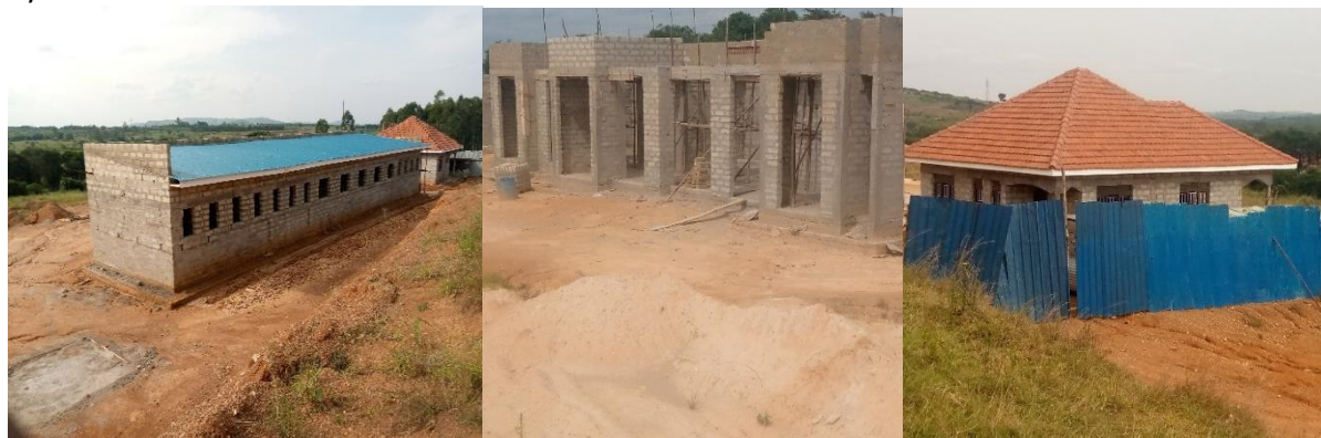
Figure 7- 1: Construction of public sanitation facility along Kampala – Mbarara road at Kiruhura
