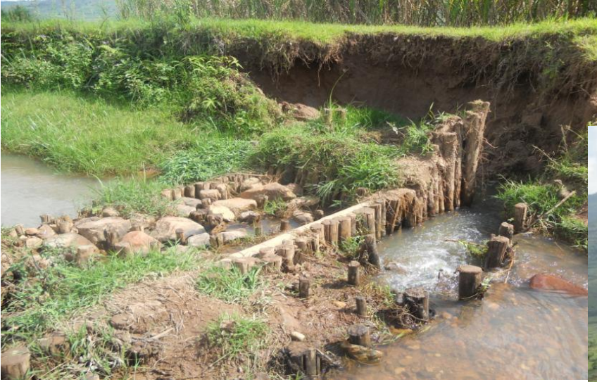
River bank stabilization
